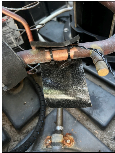
Figure 5- Applying Wrap to Sensor
